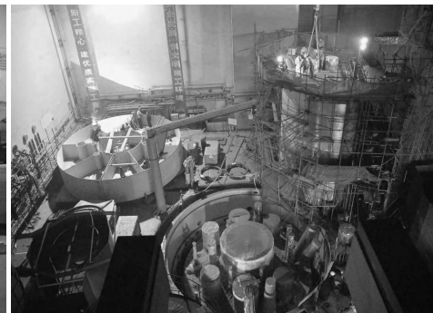
Erection of reactor vessels
