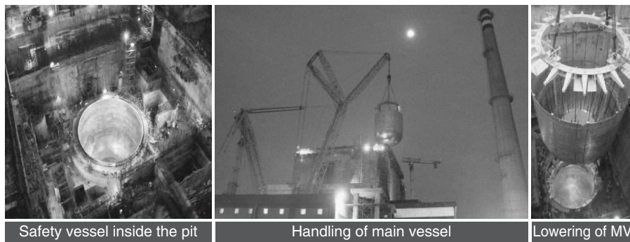
Figure 21.26 Erection of safety vessel and main vessel.
