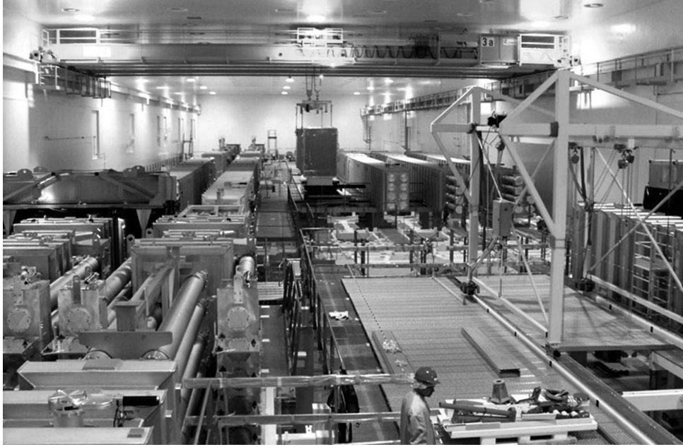
Figure 37.4 General view of the Laser Mégajoule laser hall, where the beam amplification structures are being assembled ( Courtesy CEA ).
