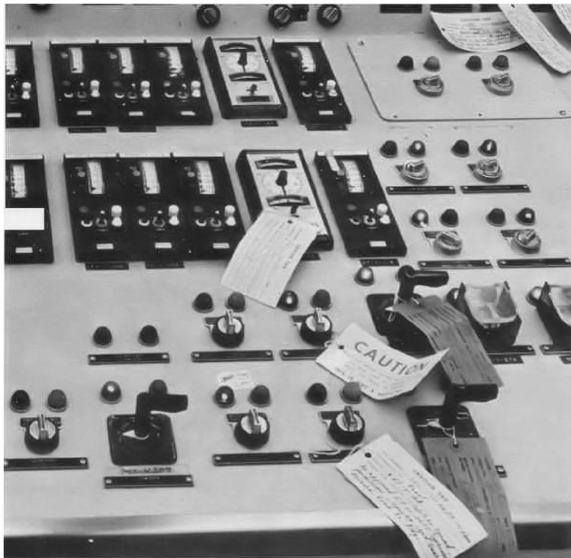
Figure 15.5 Part of the console of TMI-2 showing maintenance tags that covered some essential indicator lights during the early stages of the accident. Courtesy of the President's Commission on the Accident at Three Mile Island.
