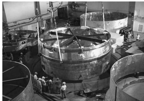
Transportation of reactor vessels
