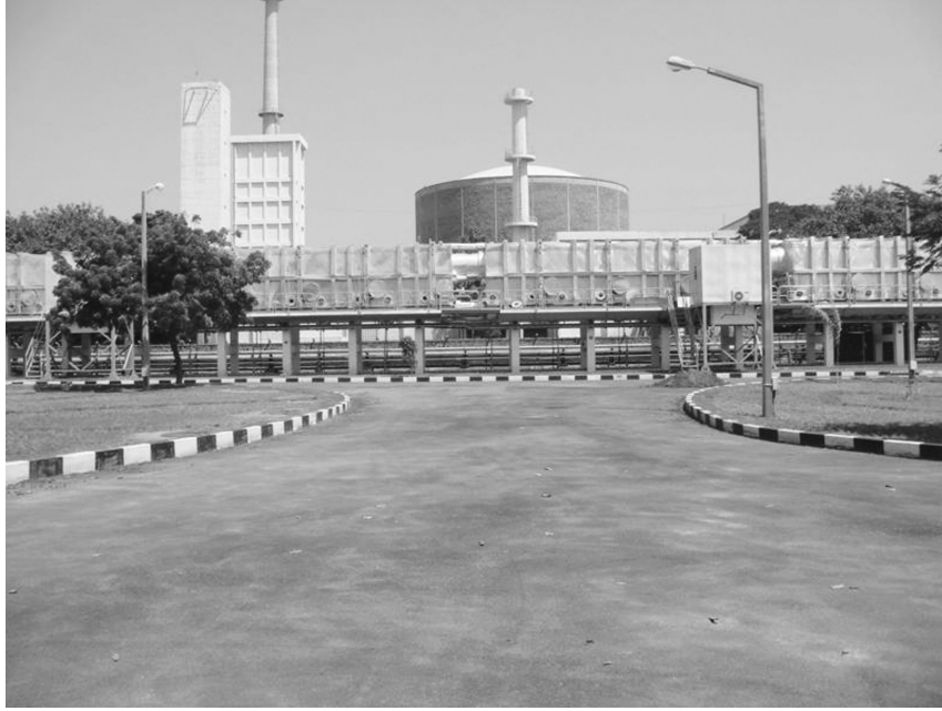
Figure 9.1 Nuclear Desalination Demonstration Plant (NDDP) at Kalpakkam (India).
