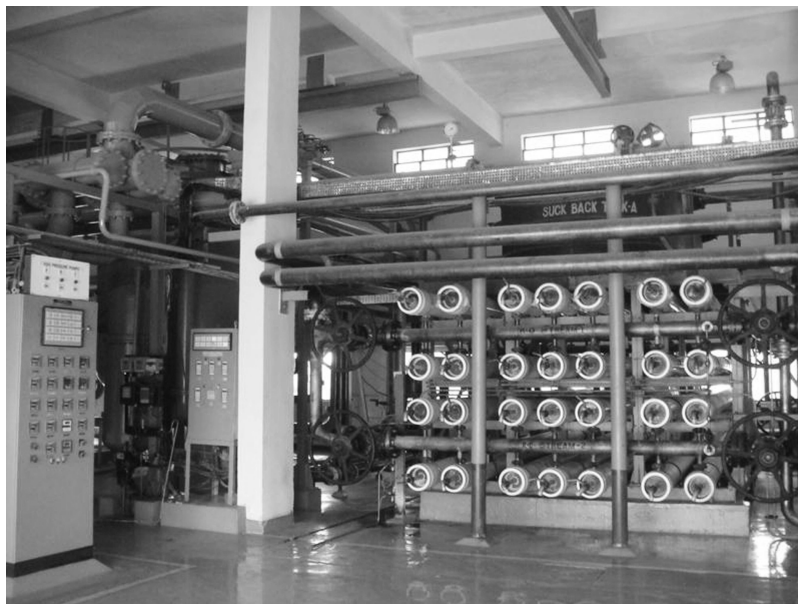
Figure 9.5 RO Section of NDDP.
