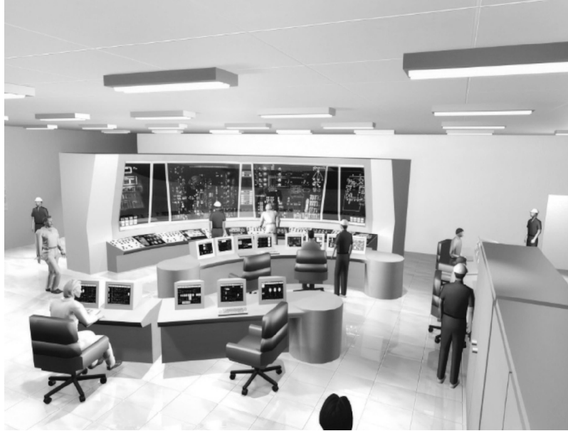
Figure 15.6 Control room of the Evolutionary Pressure Reactor (EPR) from Areva, a Generation III+ PWR reactor. The control room has separate working areas for reactor and turbine operators, shift supervisor, as well as systems and screens to show a global plant overview. Courtesy of Teollisuuden Voima Oyj (TVO), Finland.
