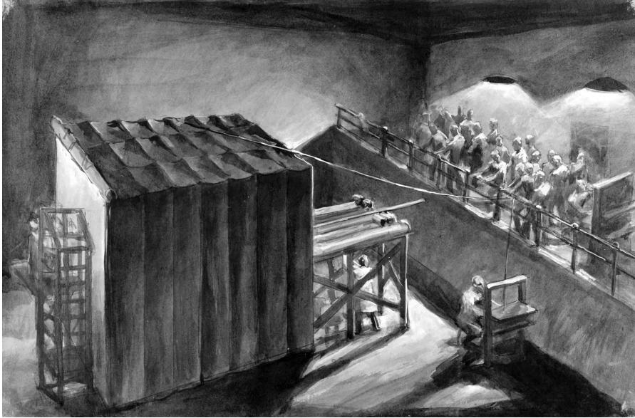
Figure 3.4 The pile showing the control and safety rods with the instrument panel and visitors on the balcony. Courtesy of Argonne National Laboratory, managed and operated by UChicago Argonne, LLC, for the US Department of Energy under Contract No. DE-AC02-06CH11357. Artist John Cadel.
