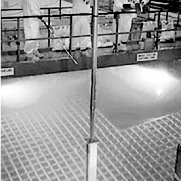
Figure 11.12 Spent fuel storage facility. Source: https://www.scientificamerican.com/article.cfm?id=japan-nuclear-renaissance .
