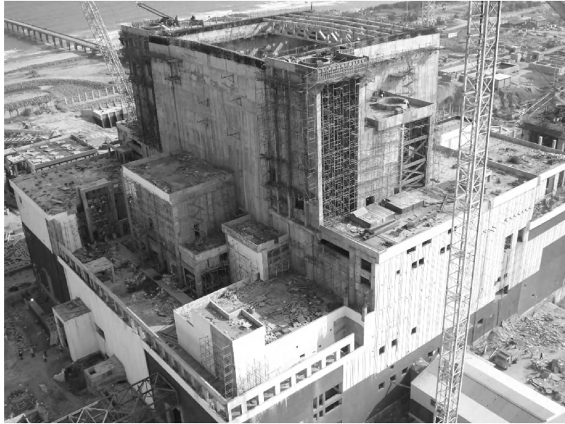
Figure 21.25 Construction of NICB.
